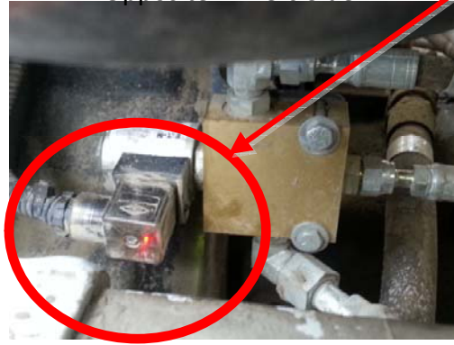
Engine Compartment Opposite Drivers Side
